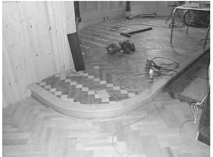
Restored Oak Chancel floor with some new nosing and risers.
